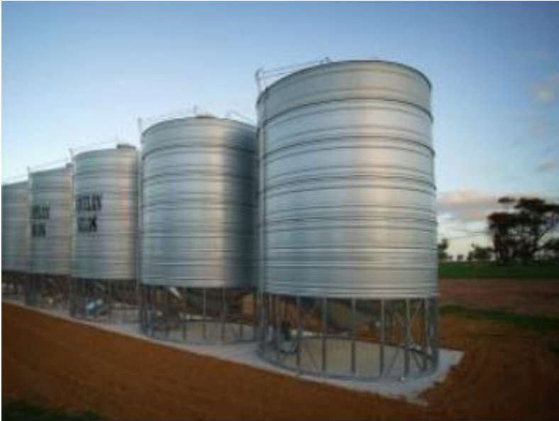
On farm grain silos. Photo courtesy of Ben White (GRDC).
